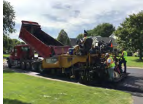
Installation of new asphalt surface
