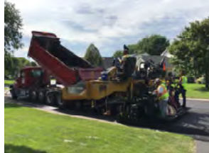
Installation of new asphalt surface
