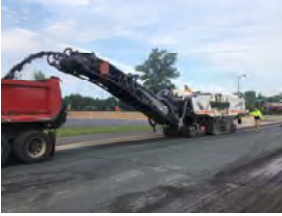
Removal of existing street surface by milling
